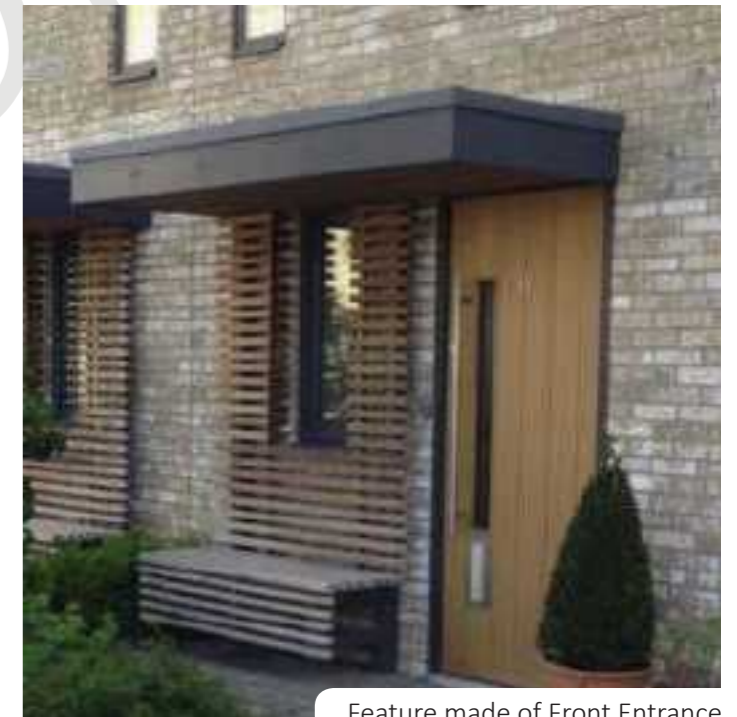
Feature made of Front Entrance
