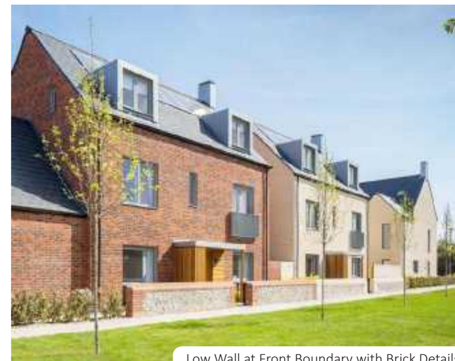
Low Wall at Front Boundary with Brick Details
