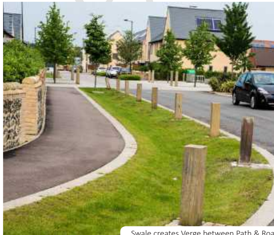
Swale creates Verge between Path & Road
