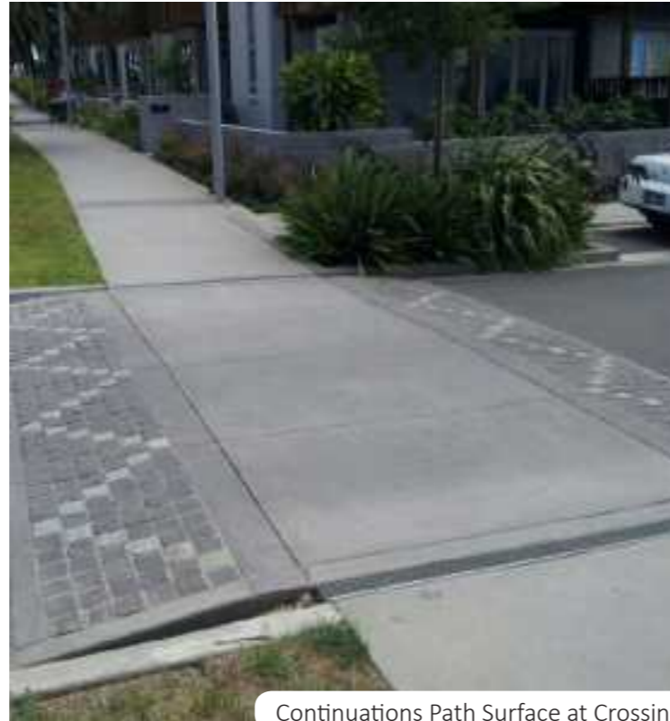
Continuations Path Surface at Crossing
